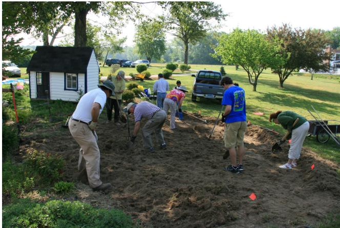
The rain garden is expected to capture all of the rain water run off from the roof and adjacent driveway. The chosen native plants will be self-sufficient once the plants are established, even capable of tolerating Maryland's typical summer droughts.
