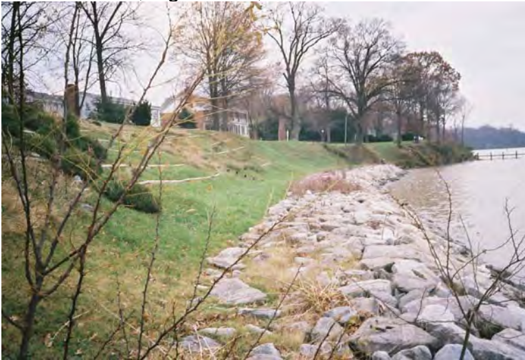
Fig. 28. A well-constructed and stable revetment. (Photo: Maryland Department of Natural Resources)
