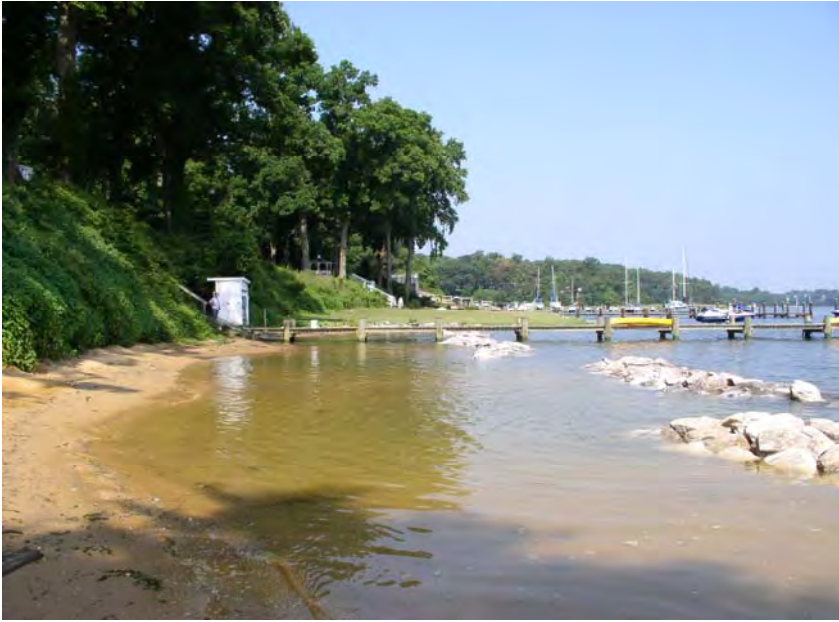
Fig. 19. Staggered and vented sill. Photo: Maryland Department of Natural Resources
