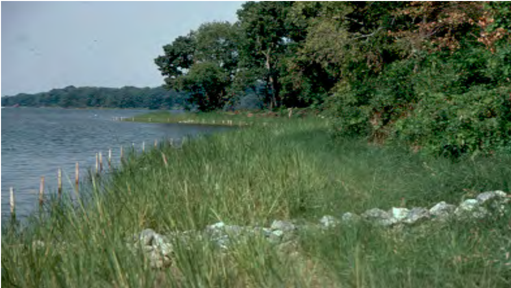
Fig. 24. Sand containment structure. Structural components placed perpendicular to the shoreline retain sand to establish a beach. These areas may also be planted. Photo: MDE
