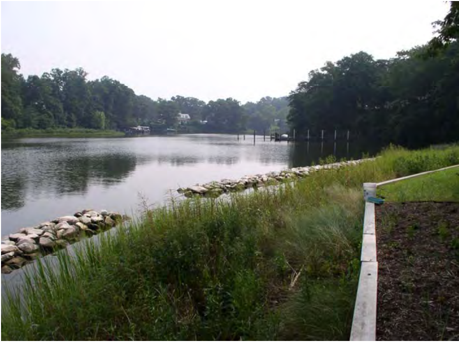
Fig. 22. Marsh and vented sill placed in front of bulkhead. (Photo: Maryland Department of Natural Resources)
