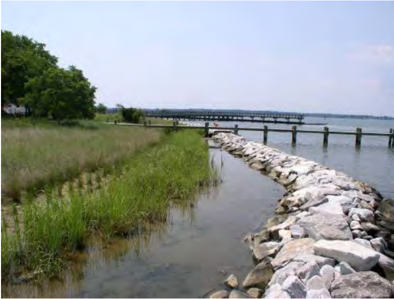
Fig. 12. Low profile sill and newly created marsh. Photo: Team Swamp, University of Maryland)
