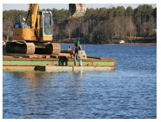
& Peterson wanted to see completed—AND they wanted to be a partner. Over the past year they installed 360 tons of concrete rubble into the shape of eleven 20-foot diameter mounds (pyramids) up to six feet tall, and six "mounds" of reef balls—three made with 31 reef balls stacked two levels high and three mounds made with 37 reef balls stacked three levels high. In all we were able to save about 50% on the true cost for this work.
