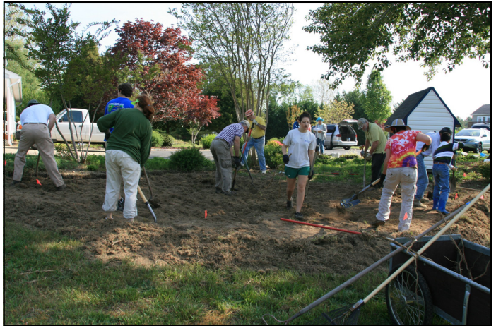
Rain Garden installation in St. Inigoes reduces polluted run-off.
